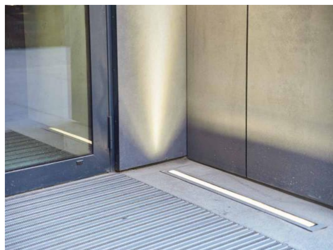
Applied luminaires: Fasad Floor LED
