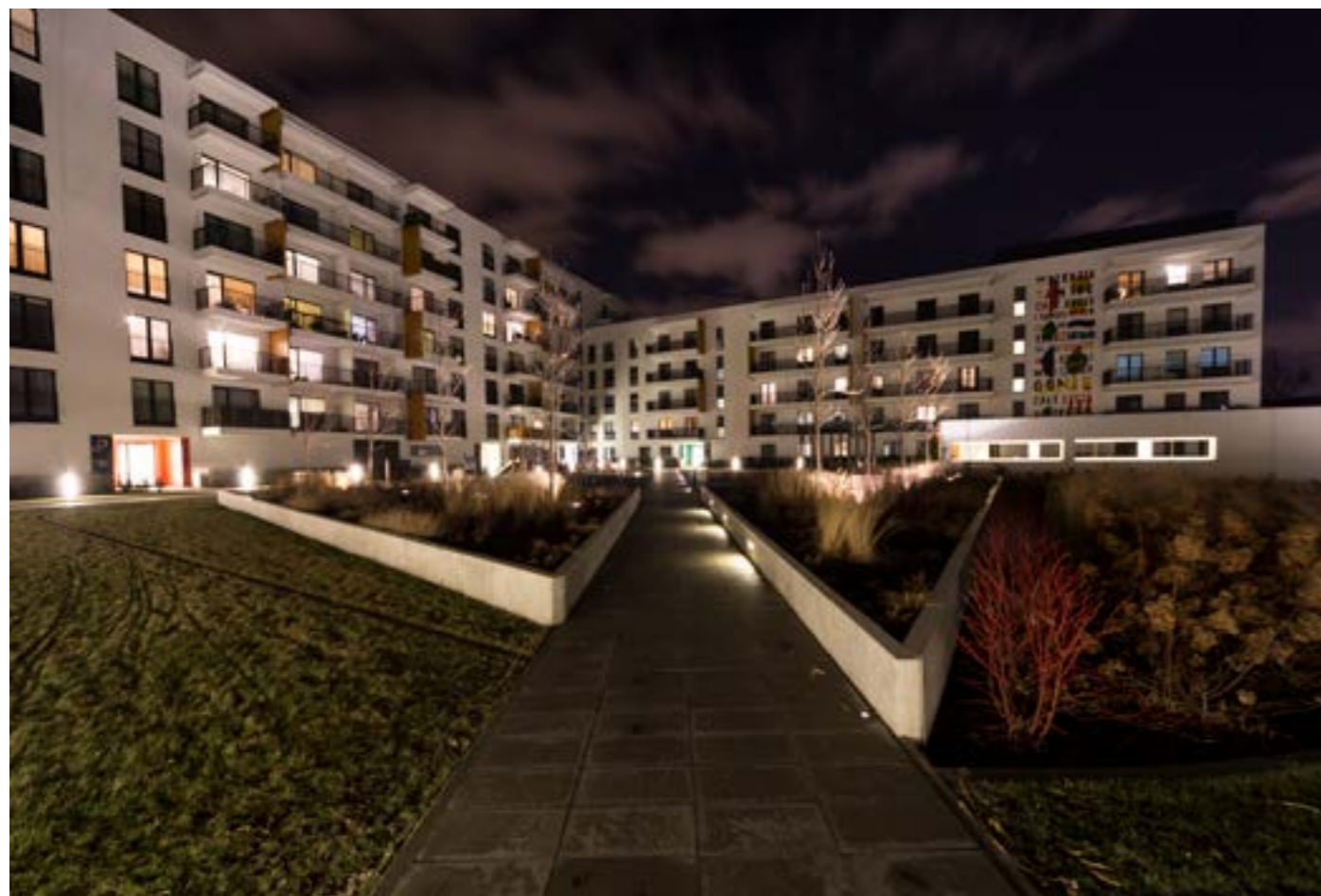
Applied luminaries: Kubik LED
