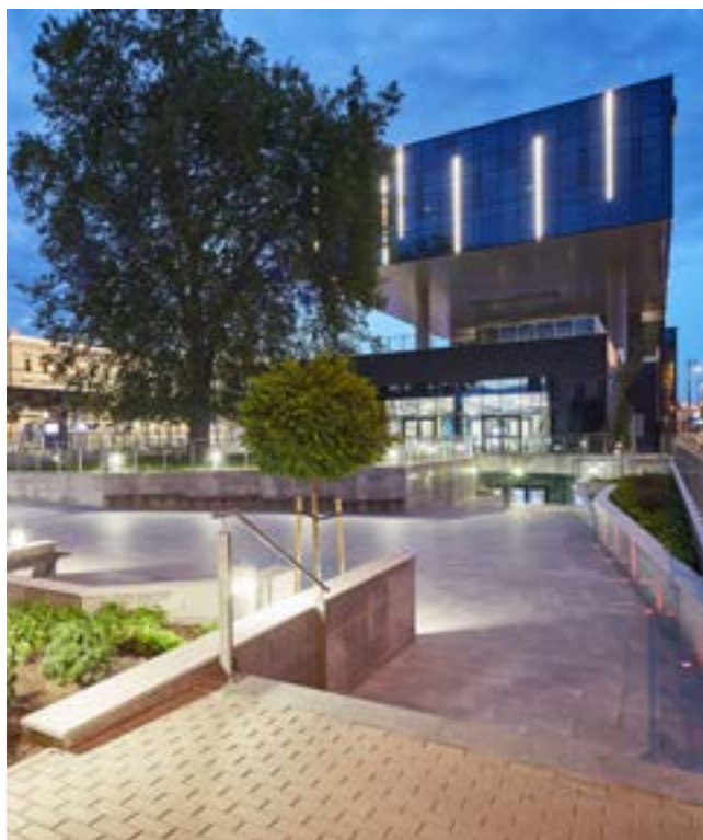
Realisation, Main Station, Bydgoszcz
