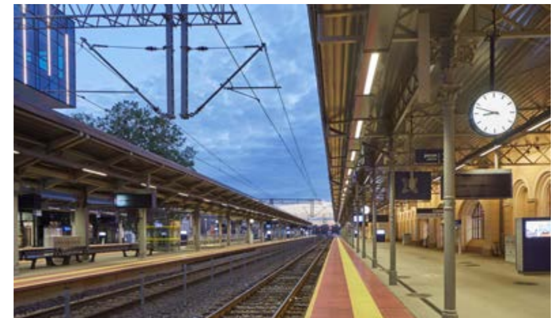
Applied luminaries: Peron Line, Lampas Out
