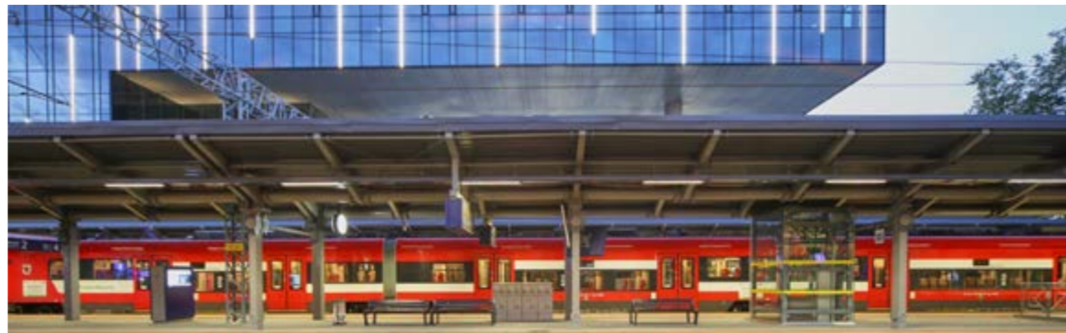
Applied luminaries: Peron Line, Lampas Out
