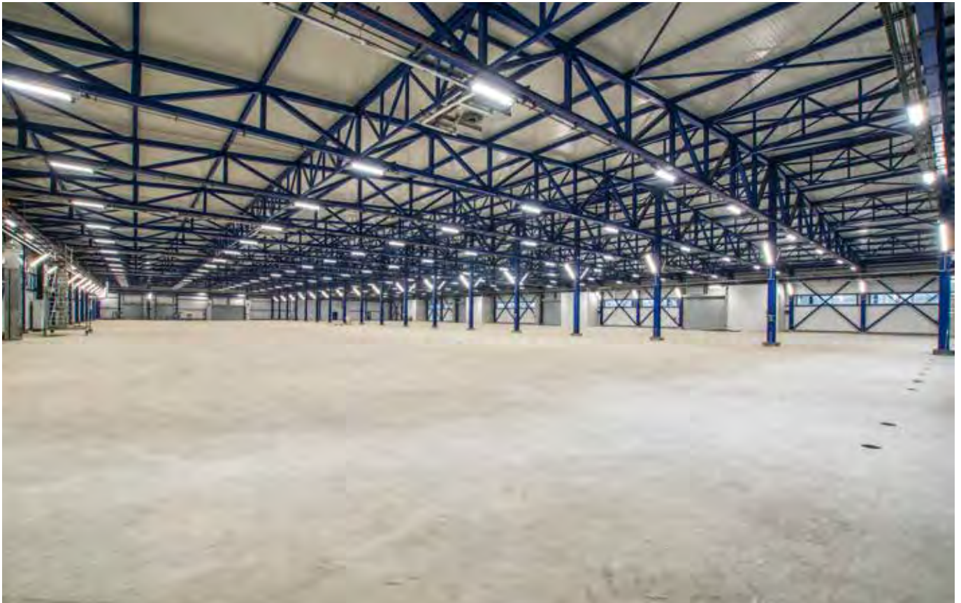
Nitrogen Plant. Puławy, Poland
