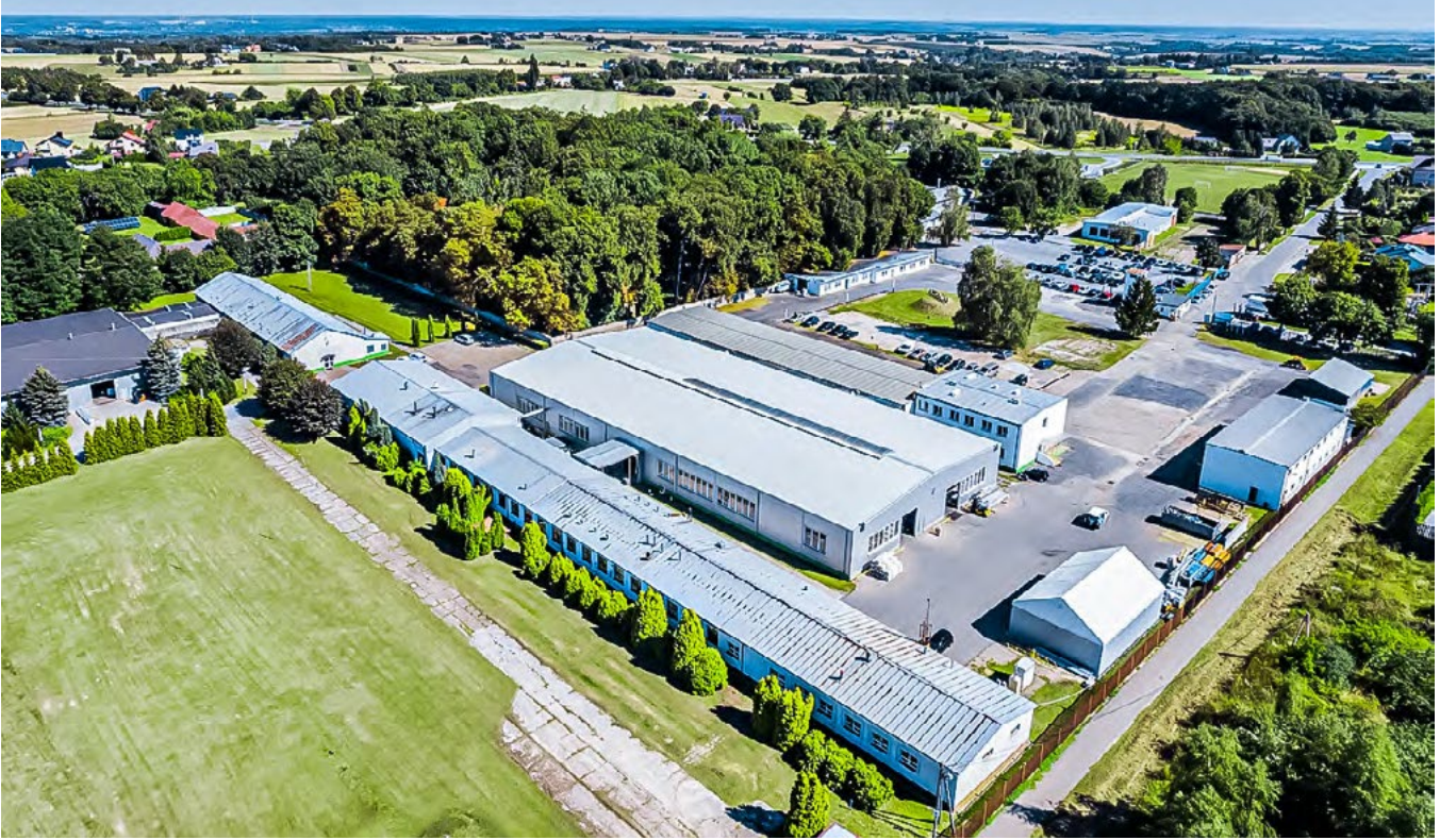
Luxiona Main Factory, Jacentow. Poland
