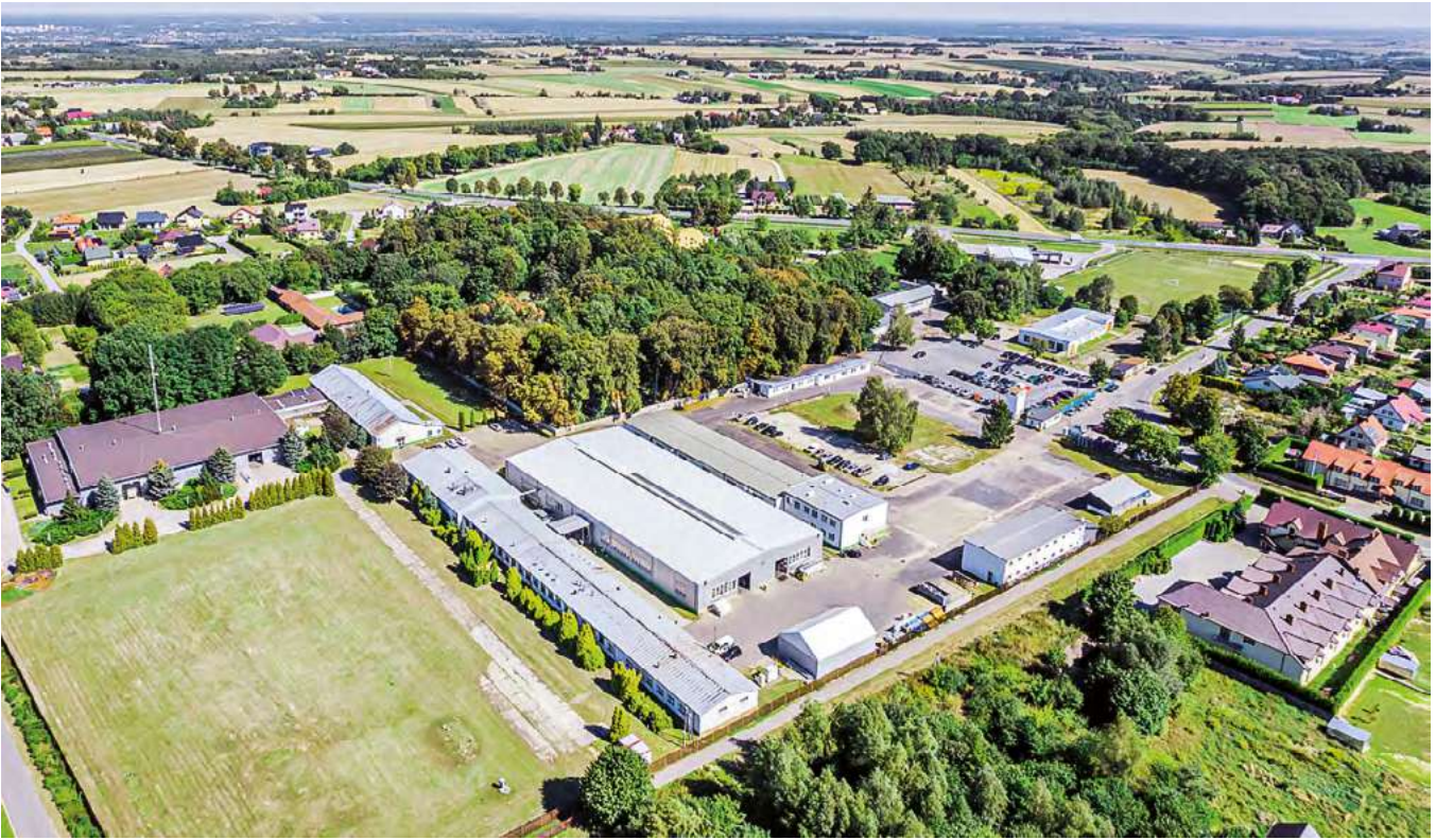
Luxiona Main Factory, Jacentow. Poland
